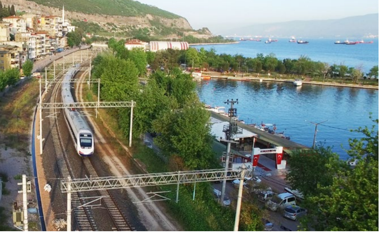
ANKARA-İSTANBUL YÜKSEK HIZLI TREN HATTI KÖSEKÖY-GEBZE KESİMİ'NİN REHABİLİTASYONU VE YENİDEN İNŞASI PROJESİ REHABILITATION AND RECONSTRUCTION PROJECT OF KÖSEKÖY-GEBZE SECTION OF ANKARA-İSTANBUL HIGH SPEED RAILWAY LINE
